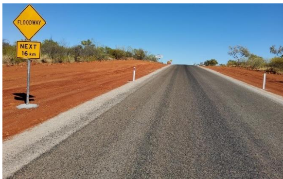
Kajabbi Road Upgrade to Seal Project complete.
