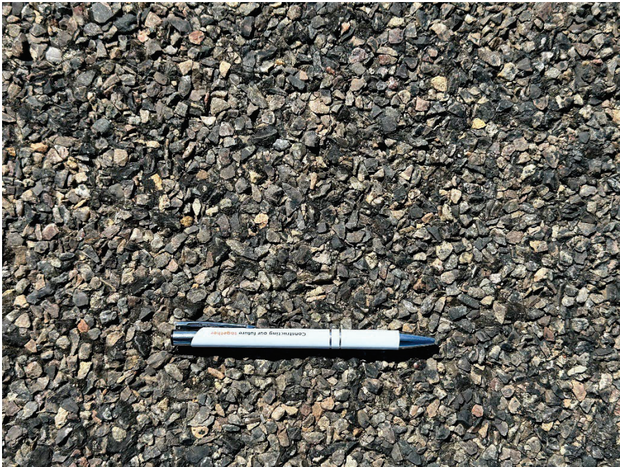
Photograph 18. Typical Taxiway C surface.
