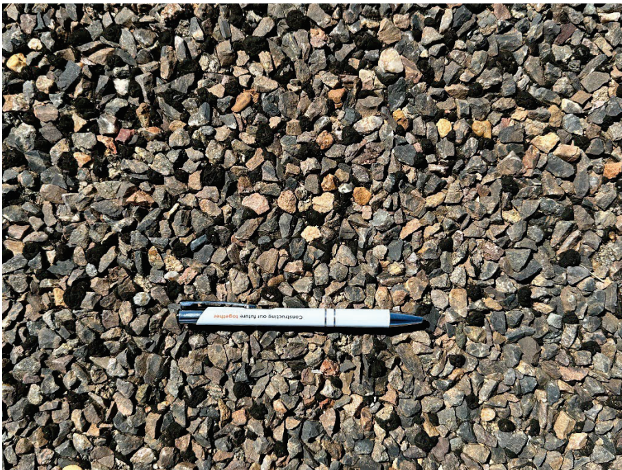
Photograph 14. Typical Runway 06/24 surface.
