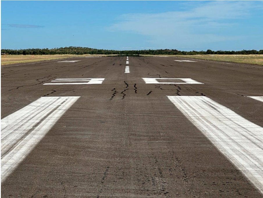
Photograph 1. General view of Runway 12/30.
