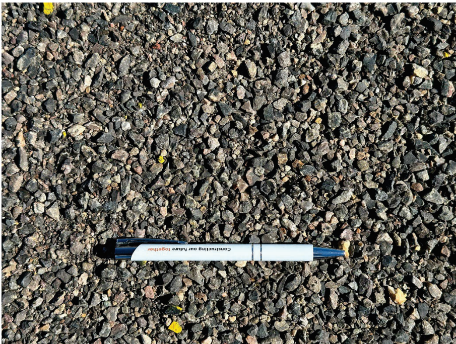
Photograph 10. Typical Runway 12/30 shoulder surface.
