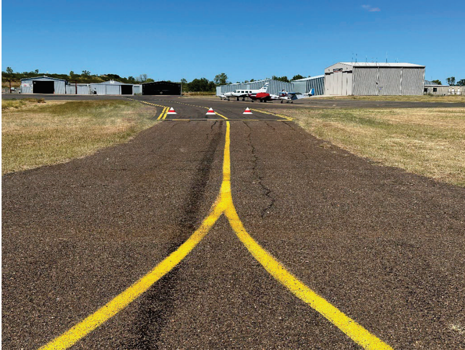
Photograph 17. General view of Taxiway C.
