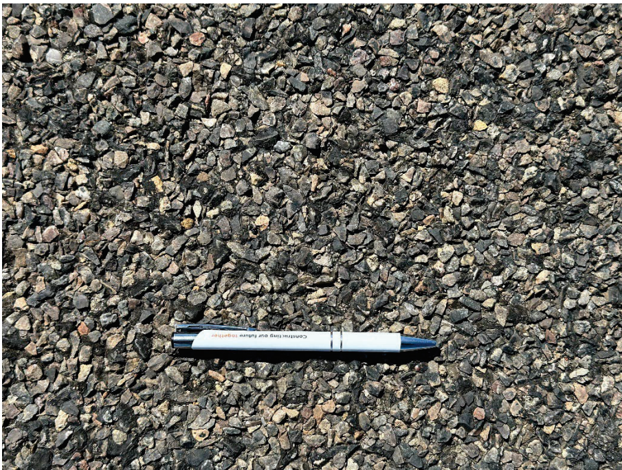
Photograph 12. Typical RPT apron surface.
