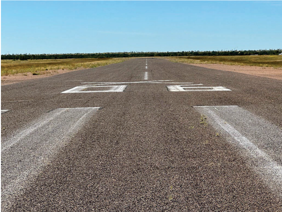
Photograph 13. General view of Runway 06/24.
