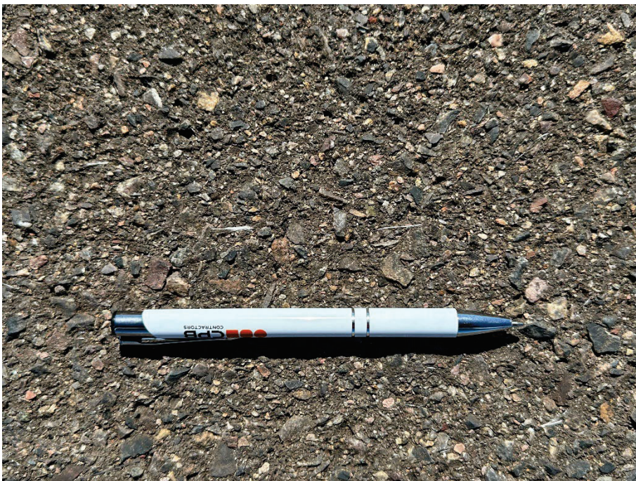
Photograph 2. Typical Runway 12/30 surface.
