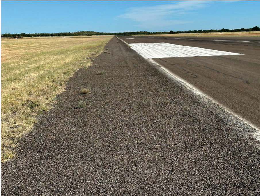
Photograph 9. Typical Runway 12/30 shoulder pavement.
