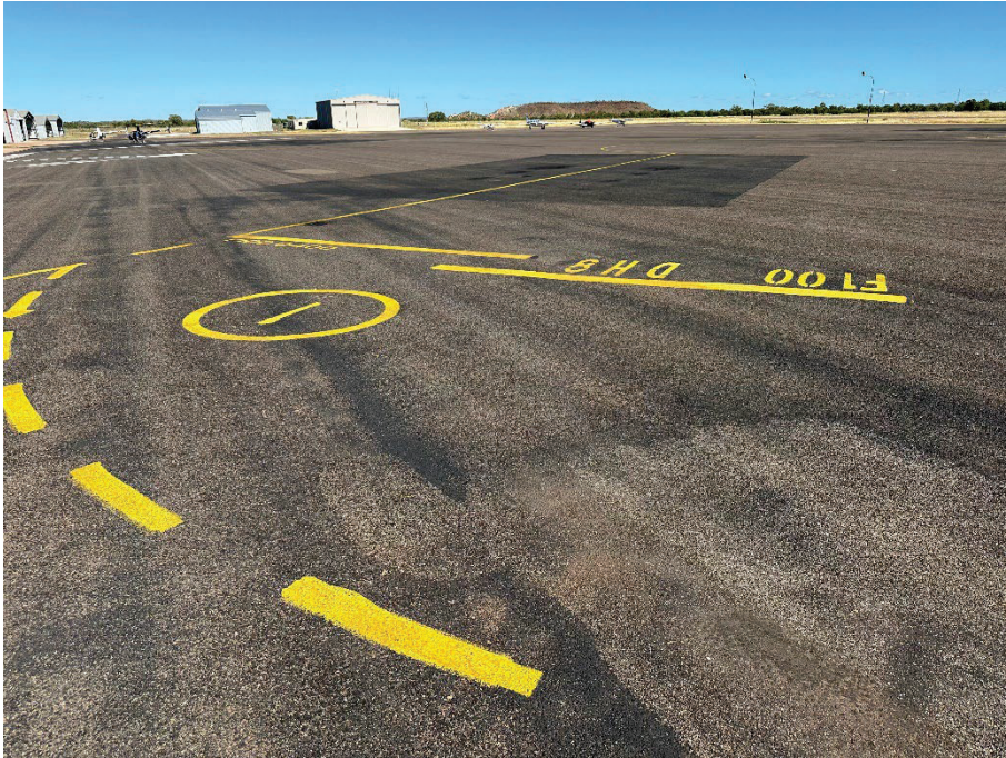
Photograph 11. General view of the RPT Apron.
