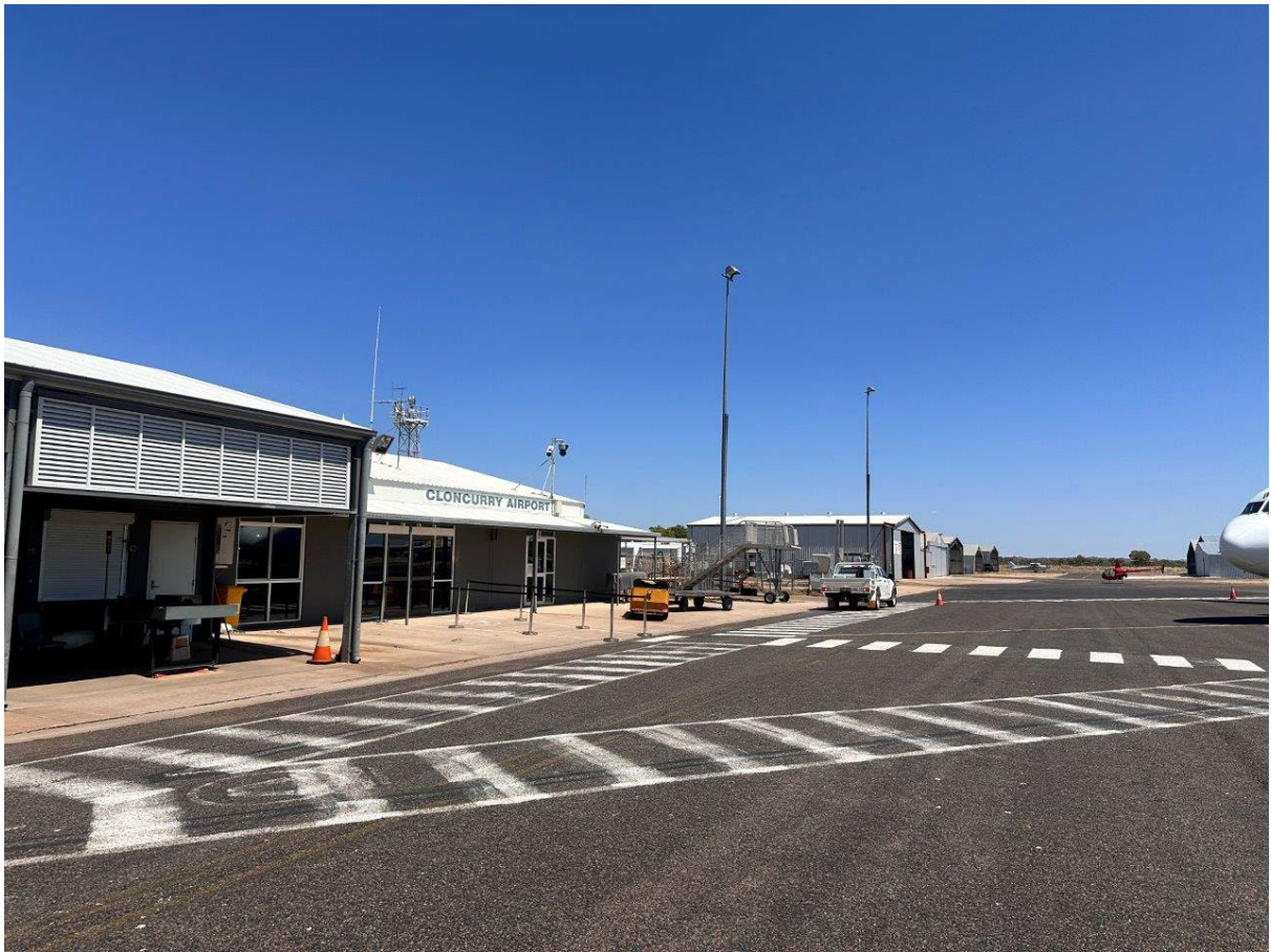
Apron Floodlight Poles (SW edge)
