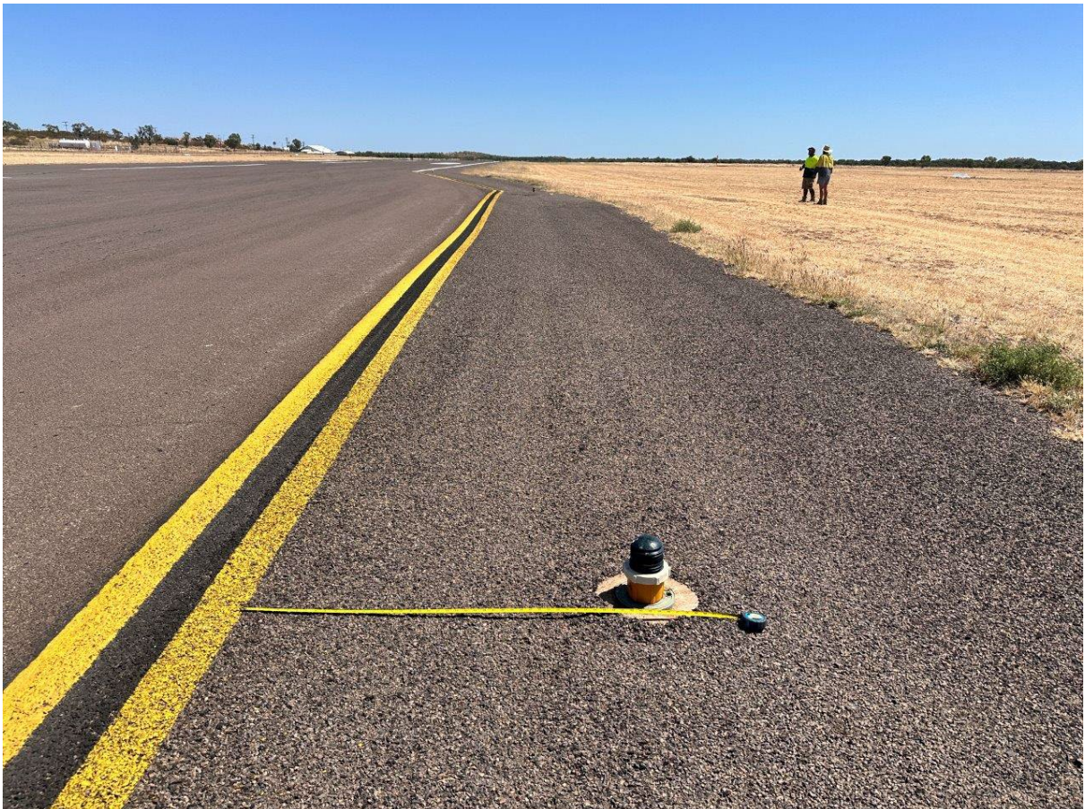
Elevated Turning Node Light
