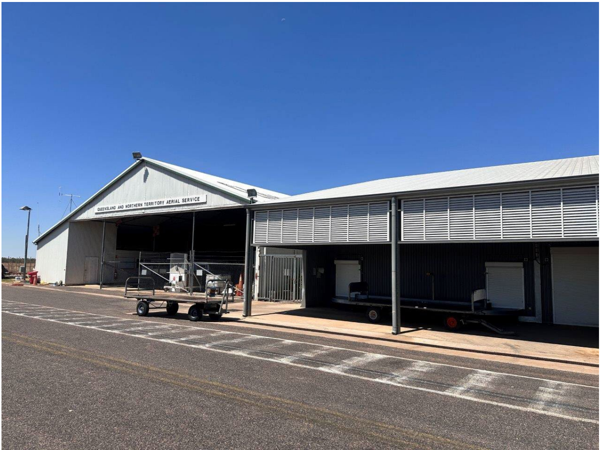
Apron Floodlight Poles (SW edge)
