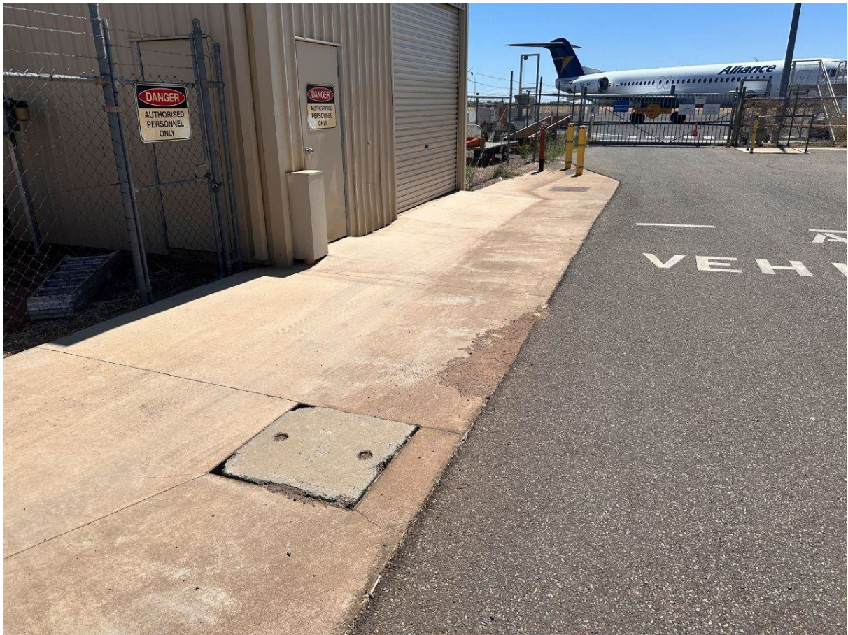
Airfield Lighting Equipment Room (ALER) – Facing NW
