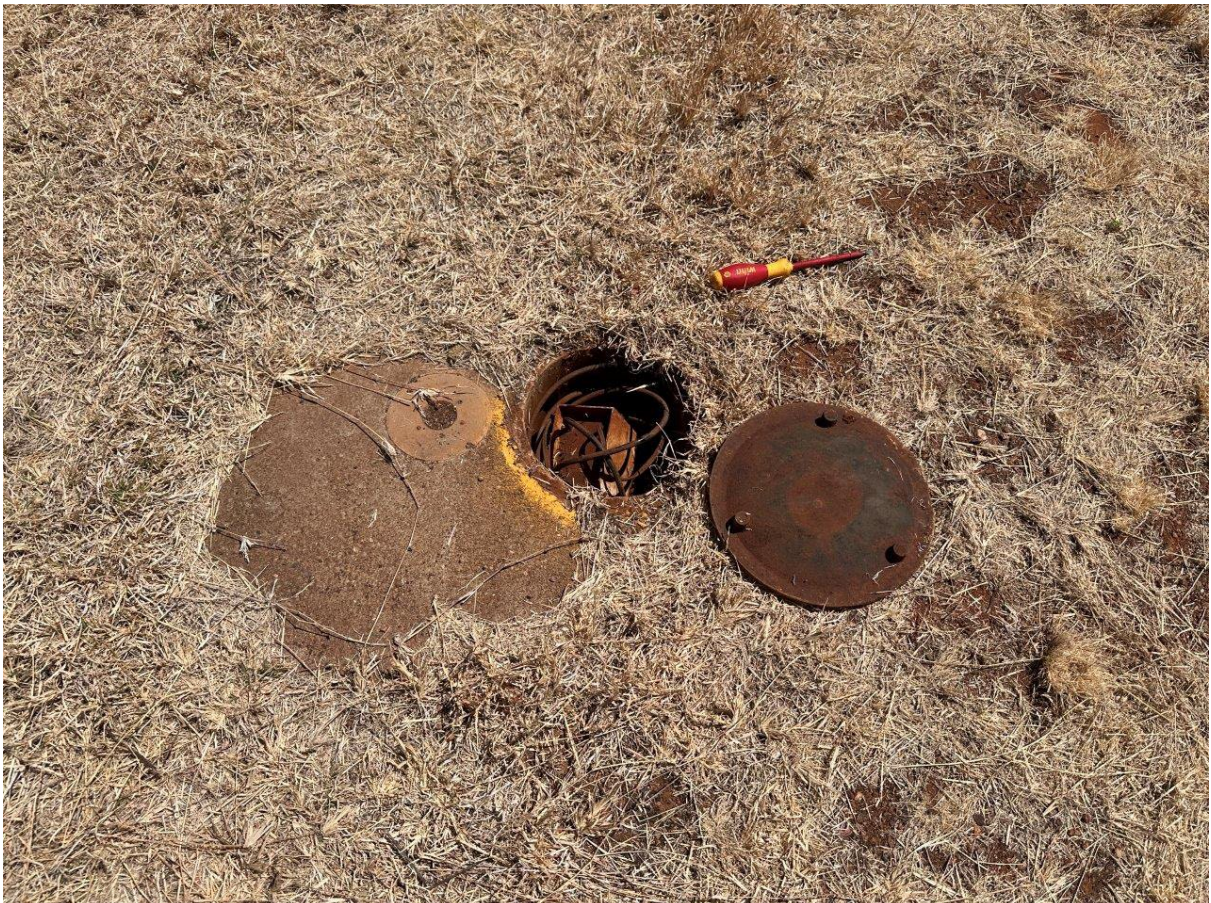
Runway Edge SIT Pit (close-up)
