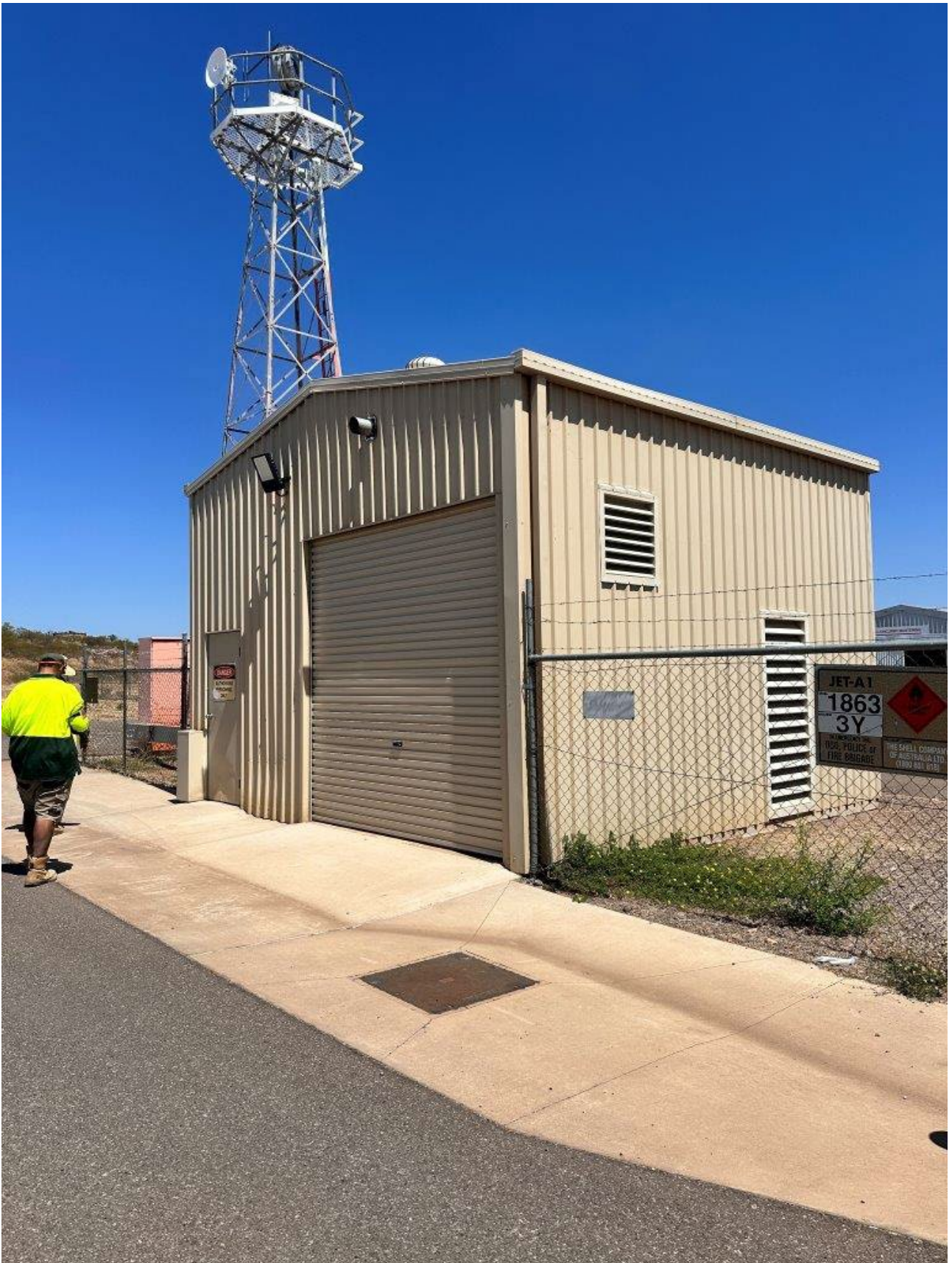
Airfield Lighting Equipment Room (ALER) – Facing SE
