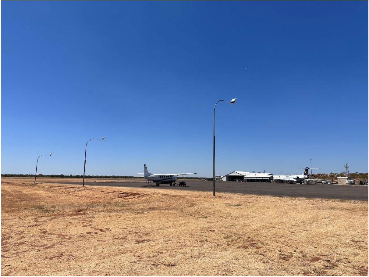
3 x Apron Floodlight Poles (NW edge)
