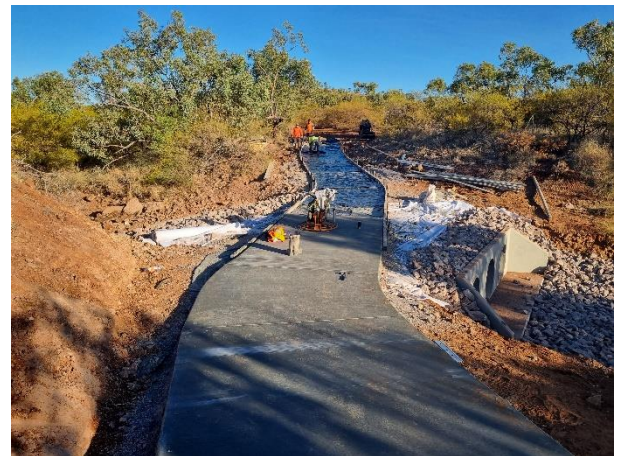
Auzscot Constructions continue work on the Path to Chinaman Creek Dam
